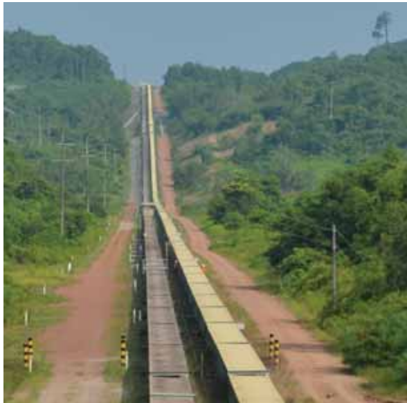
Typical overland conveyor
